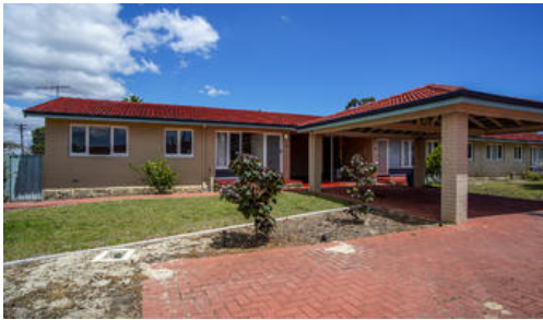
Unit 8, 72 Amberton Ave, Girrawheen
