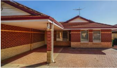
Unit 10, 268-272 Wharf St, Queens Park
