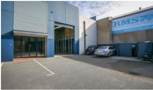
Unit 7, 10 Franklin Lane, Joondalup
