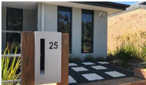
25 Stanbury Crescent, Ellenbrook
