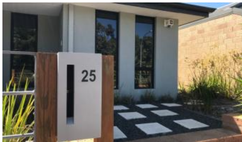
25 Stanbury Crescent, Ellenbrook
