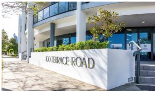
Unit 52, 100 Terrace Road, East Perth
