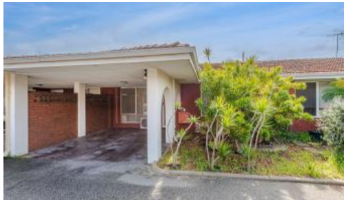
Unit 2, 194 Edward Street, Osborne Park
