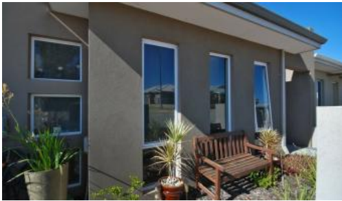
11 Pymore Crescent, Butler
