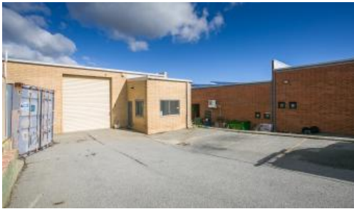
Unit 1, 22 Dellamarta Rd, Wangara
