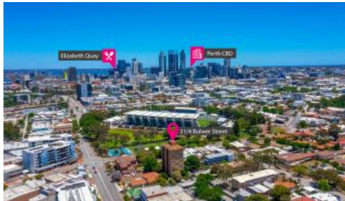
Unit 31, 4 Bulwer St, Perth
