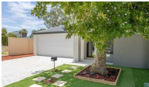
1B Wickens Street, Beckenham
